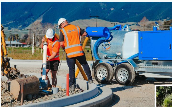
Non-destructive hydro excavation is extremely safe and productive for many uses including:
